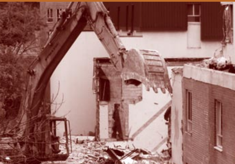
Don Mount Court demolition
